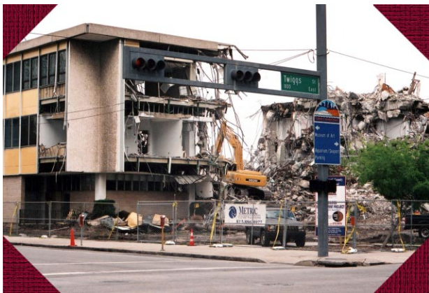
Edgecomb demolition began in spring 2001.
