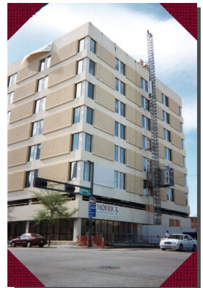
Twigg Street building was renovated in 2000.
