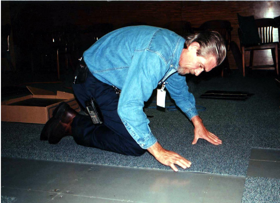
Gordon Perkins, from Court Facilities restores carpet in Courtroom 1.
